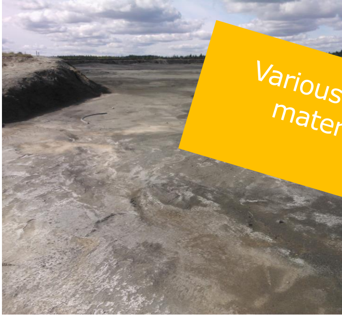
Tailing pond in Hitura Mine
