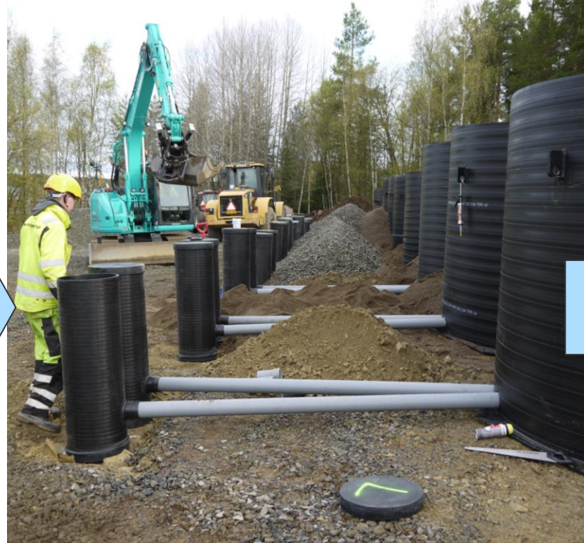
PILOT TESTING IN FIELD CONDITIONS
